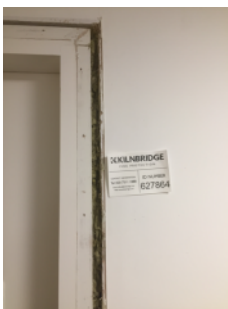
4th floor staircase door frame during fire stopping
