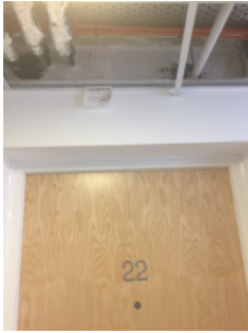
Inner layer fire stopping above flat 22
