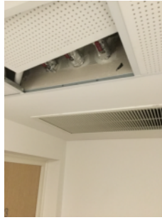
Fire stopping into the smoke shaft by flat 73.
