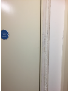
5th floor riser cupboard door frame completed fire stopping.
