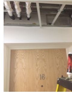
Fire stopping in progress above Flat 16 entrance door.
