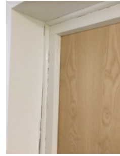
The architrave has been removed and fire stopping carried out.
