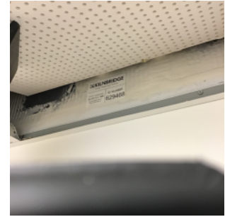
Version 8 Fire stopping 5th floor electrical riser
