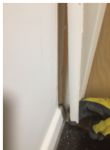
Flat 47 entrance door example of completed fire stopping
