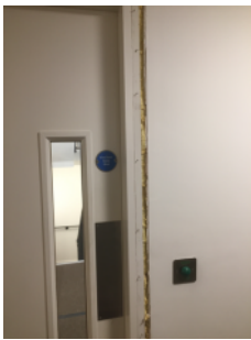
4th floor staircase before fire stopping
