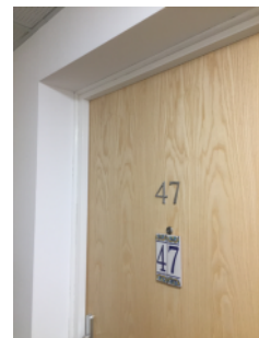
Flat 47 quadrant replaced.
