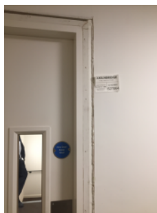
4th floor staircase door frame fire stopping
