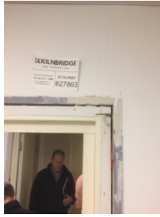
Example riser cupboard door prepared fore fire stopping.
