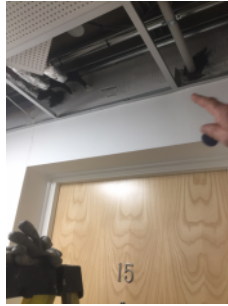
Fire stopping completed above Flat 15
