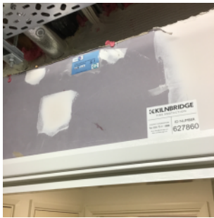
Version 8 Evidence of fire stopping in 5th floor electrical riser
