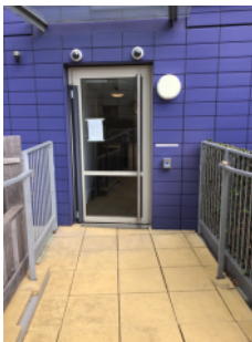
Communal terrace access door
