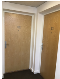
Typical main flat entrance doors
