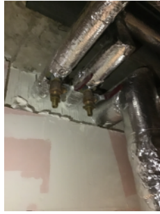
Example of good fire stopping within riser cupboard, 4th floor.
