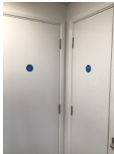
Riser cupboard doors with keep locked shut signage
