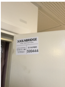
Evidence of recent fire stopping.
