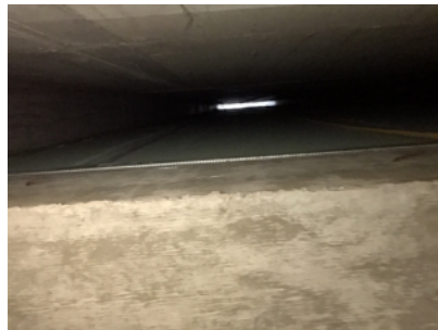
Void at rear of pump room, lower ground floor to roof.
