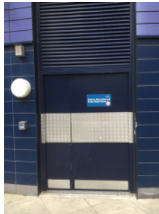
The bin store was secure at the time of the visit
