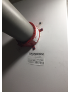
Evidence of remedial fire stopping
