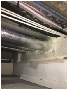
Good fire stopping above lobby door, 9th floor.
