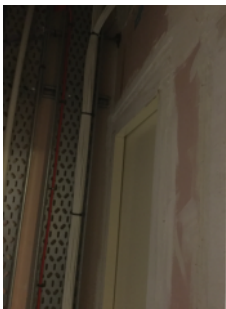
Riser cupboard door, sixth floor.
