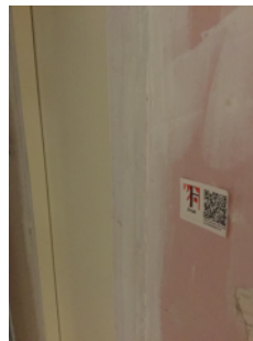
Fire stopping around the door frame, riser cupboard sixth floor.
