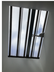
Corridor AOV on 10th floor
