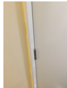
Evidence of that the architrave has been removed.
