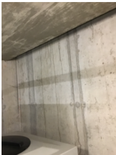
Void at rear of pump room, lower ground floor to roof.
